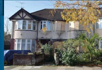
Lot 116 – March Terrace fire damaged house
